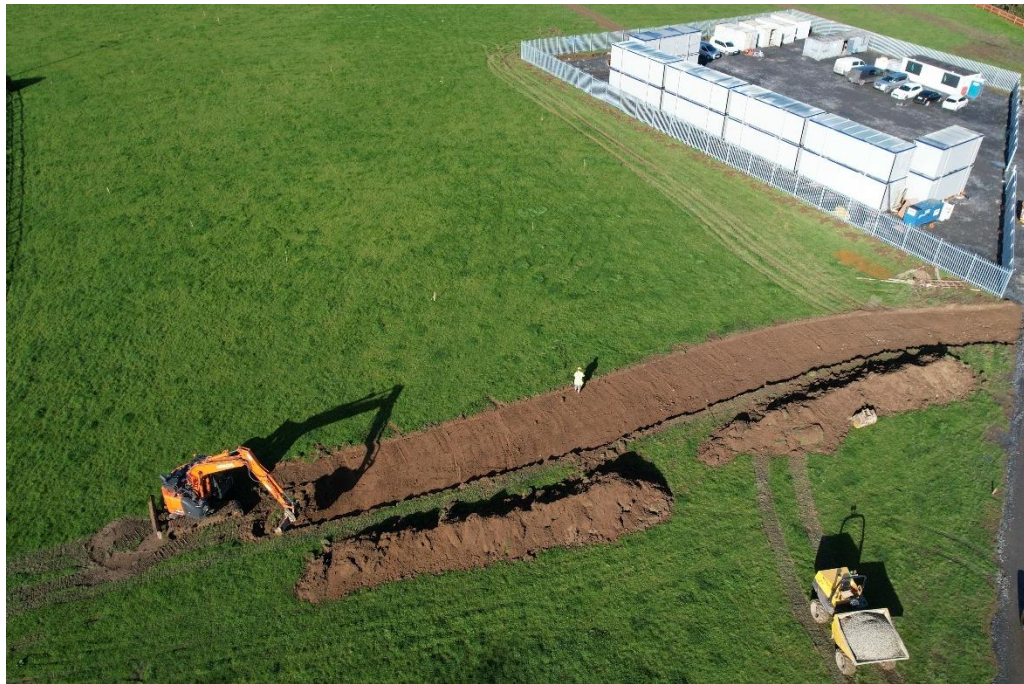
Plate 12 Aerial view of topsoil stripping for haul road, 24E0045ext.
